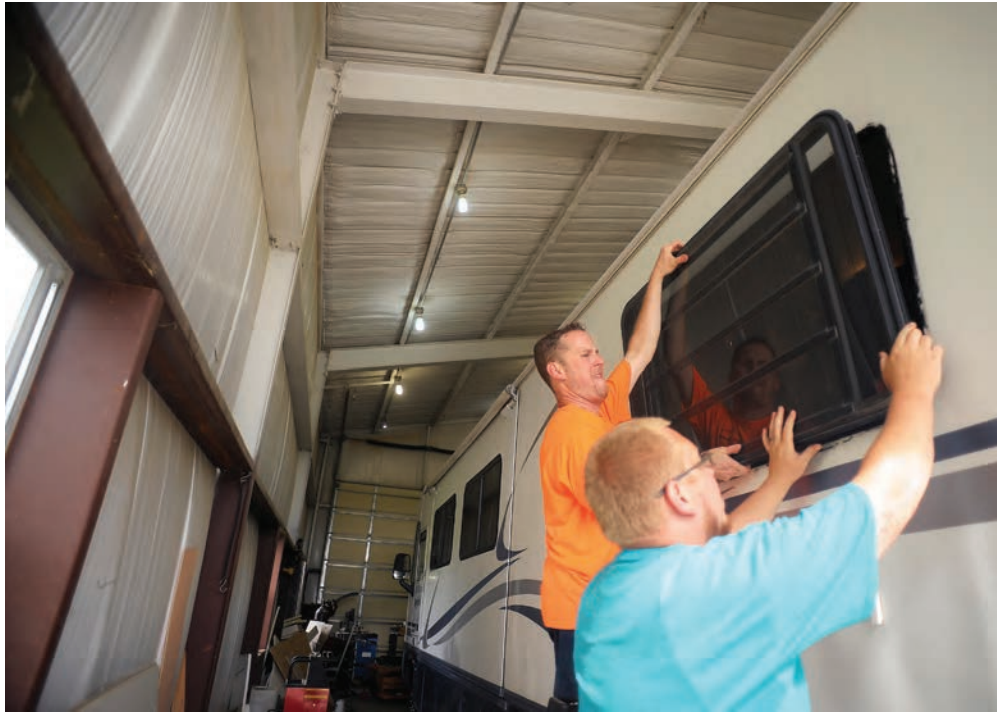
Mike Suto and Jimmie Hughes work on installing a window in a refurbished RV at Green Country RV Doctor. The bulk of the Green Country RV's business comes from general maintenance of RVs, such as fixing plumbing leaks and toilet problems, lights, and electrical. About 15 percent is customizing and remodeling RVs. Another 10 percent focuses on mechanical servicing of mobile units such as oil changes. The rest comes from the repairs and maintenance of the rubber roofs and winterizing RVs.
